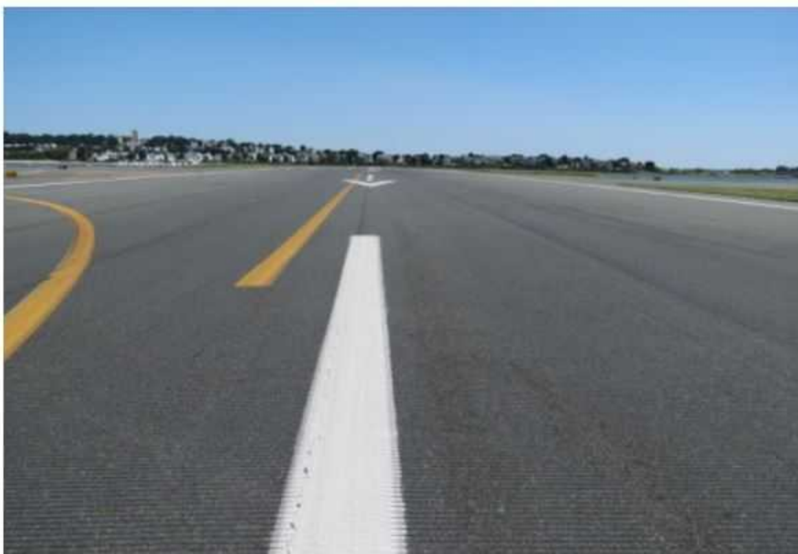
(Above) This is an aerial shot of the Boston-Logan Airport showing where StellarFlex FR™ was laid, and (below) are images of the finished pavement showcasing how great the grooving looks after 10 years. It is straight and true with no rutting and deformation.
